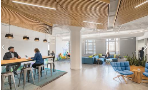
Wood louver ceiling
